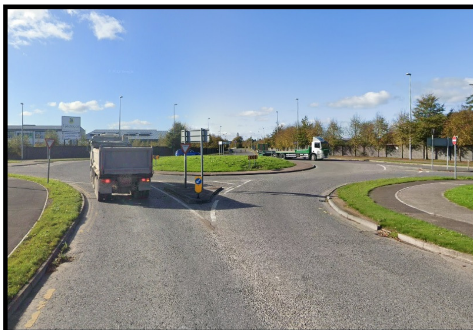
Figure 2.3 – Adjacent Roundabout, View West (Google)
